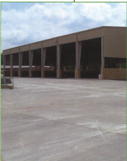
Significant modifications were made to the digestion and storage facilities to meet the needs of the expanded facility.
