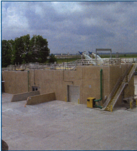
The new headworks at the facility is designed to provide fine screening, grit removal and preaeration of influent wastewater.
